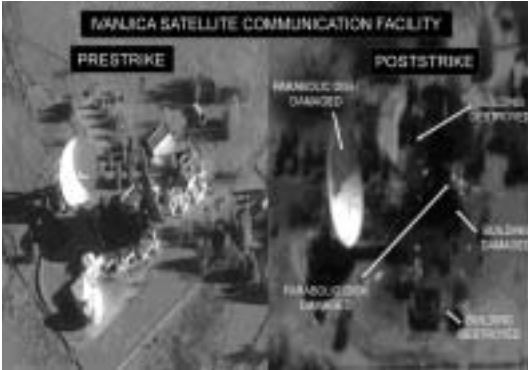
This picture, courtesy of NATO, documents the damage to the satellite antenna and the surrounding infrastructure at Ivanjica satellite ground station.
